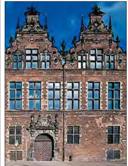
The Arsenal seen from Targ Węlowy
