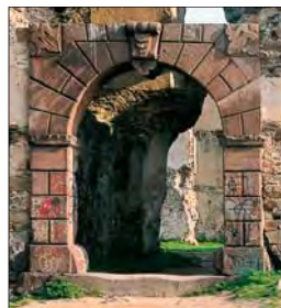
Ruins of the Baroque Bishops' Palace at Bodzentyn
