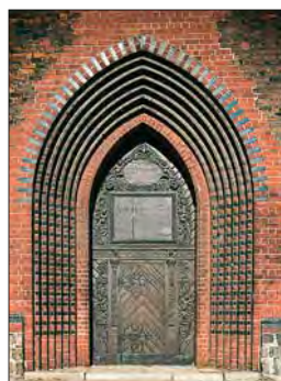
Portal of the Cathedral of St James
