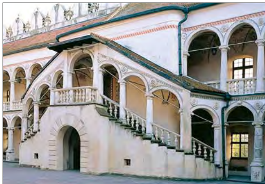
Staircase in the courtyard of Leszczyński Palace in Baranów Sandomierski
