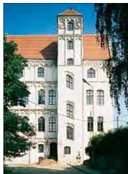
Loitz House, once the home of a family of bankers
