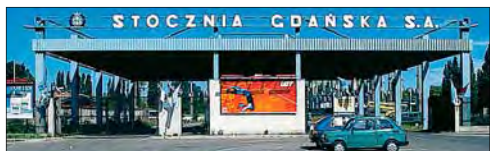
Main entrance to the Gdańsk Shipyard
