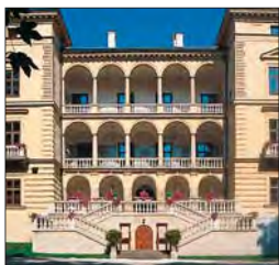
Decjusz Villa from the garden, the arched loggia flanked by towers
