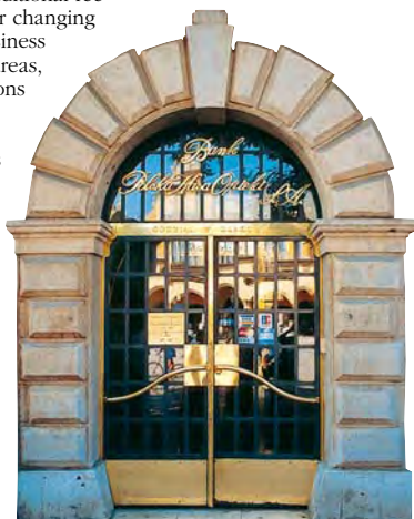
Entrance to the bank PKO in Cracow
