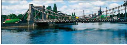
Grunwaldzki Suspension Bridge
