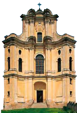
Baroque façade of the Benedictine church in Drohiczyn
