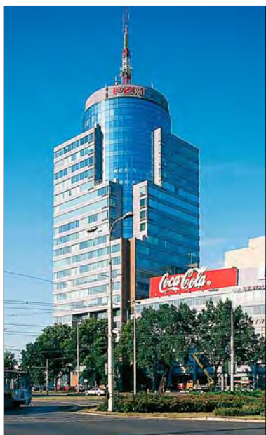
The Pazim, the tallest building in Szczecin
