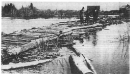
Fig.3 Corduroy bridge across Whitemouth River
