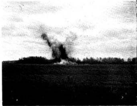
3-9. A dugout is being blasted out. W. Happychuk
