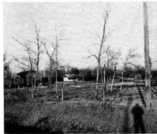
3-10d. Showing the buildings of a smaller livestock farm found in the Vita area.
