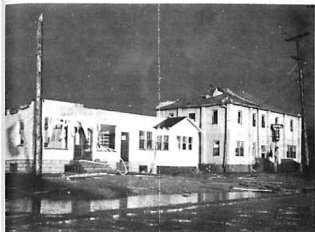
Badly damaged were Vita Bakery (left) and Vita Hotel (right), both operated by M. Kadyniuk and sons. The bakery lost its roof and the inside appeared to have been turned upside down. The hotel lost most of its windows and the interior was partially wrecked.
