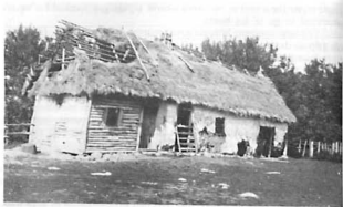
An abandoned pioneer house. Note construction.
