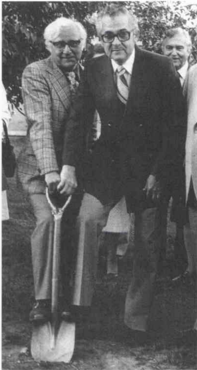
Breaking ground for the annex, 1979
