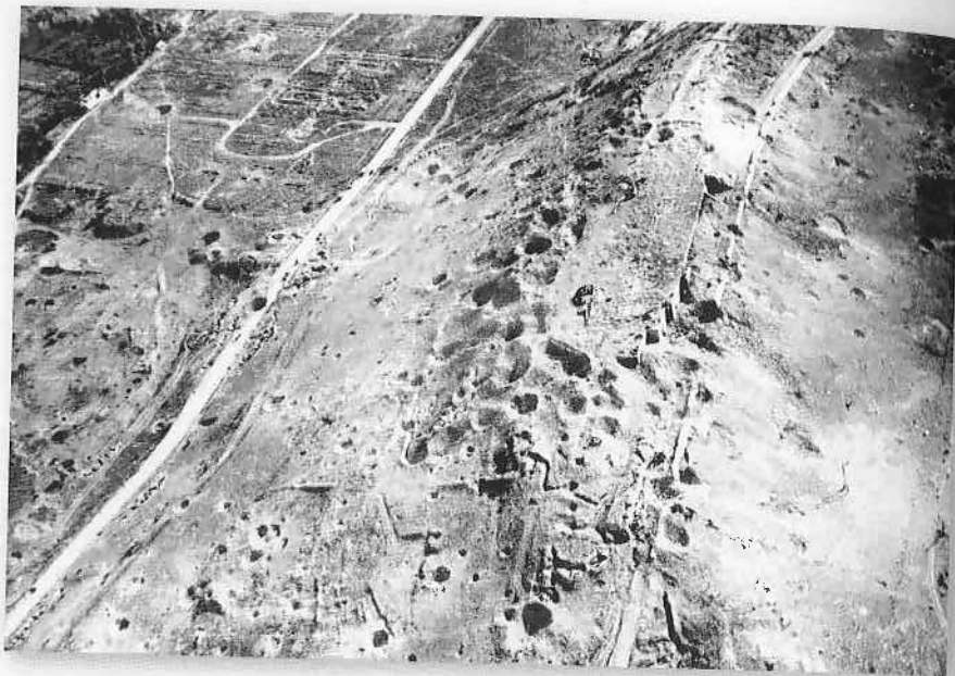
Aerial view of Coastal Battery 30 after the fighting. The roof of Turret No. 2 has been blown off. Note the large craters from multiple super-heavy artillery rounds. (Ted Nevill, TRH Pictures)
