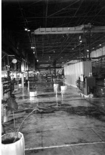
Figure 7.11. The turbine hall, December 1987. (Photograph: R F Mould.)
