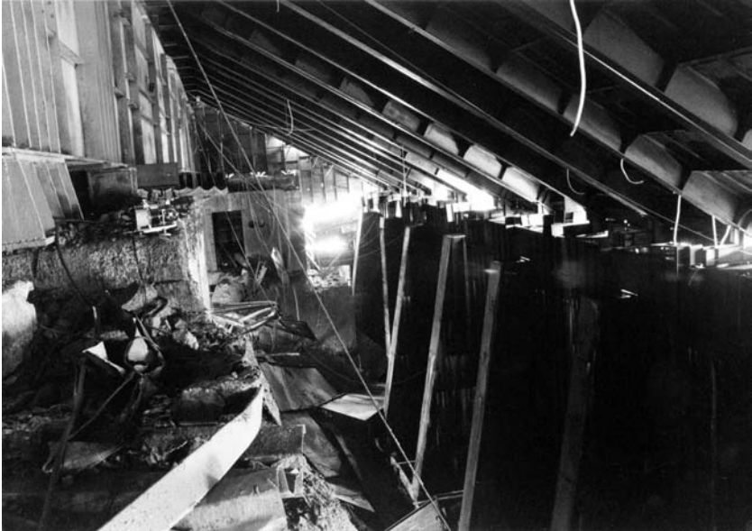
Figure 7.5. Inside the Sarcophagus near the cascade wall, 1996. (Courtesy: Chernobylinterinform.)
