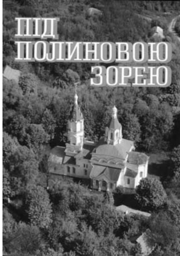
Figure 20.7. Aerial view of the church of St Eliah in Chernobyl town. (Courtesy: R Omelyashko.)
