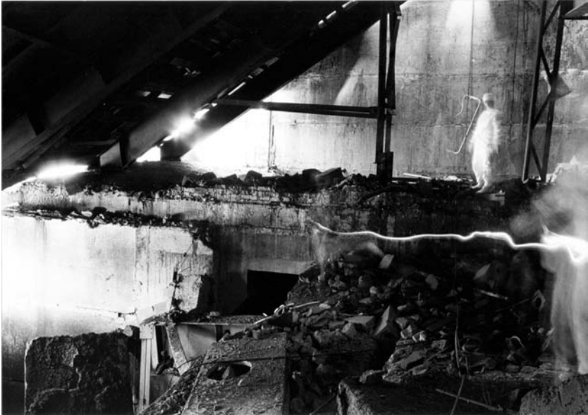
Figure 7.6. Inside the Sarcophagus near the cascade wall, 1996. (Courtesy: Chernobylinterinform.)
