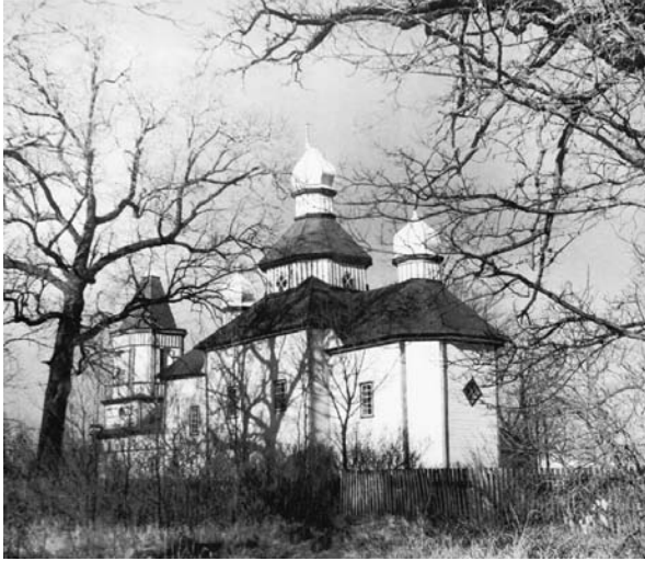
Figure 20.9. 17th century wooden church in the village of Tolsty Les. It was totally destroyed by an accidental fire on 24 April 1996. (Courtesy: R Omelyashko.)
