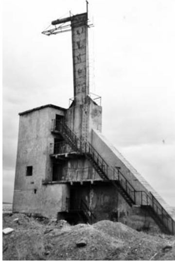
Figure 4.6. Building at Ground Zero which was used to monitor radiation effects: colloquially known as the Goose Neck , May 1999. (Courtesy: V Mouchkin.)
