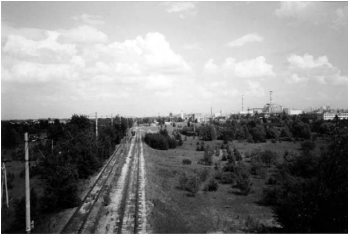
Figure 14.12. View of the power station from the bridge over the railway line at Yaniv, 1998. This line was so contaminated by the accident, see Yaniv in figure 14.9 within the beta contamination boundary of 6000 \text{ kBq/cm}^2 . The railway was so badly contaminated in April 1986 that it could not be used for evacuating the population. (Photograph: R F Mould.)
