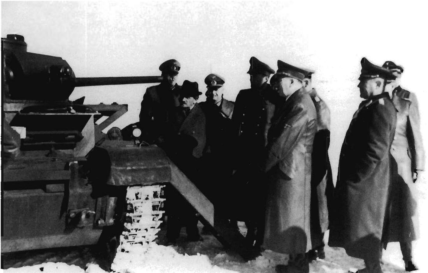
Hitler and the dignitaries of his party inspect several German and Russian tanks at Zaporozsche. The tank in the picture is a Panzer III, equipped with a 5cm main gun. A longer barreled gun of the same caliber was in extensive use already, although even the improved gun was inferior to both the 7.6cm gun of the T-34 and the L42 (7.5cm) gun of the Panzer IV (Credit National Archives)
