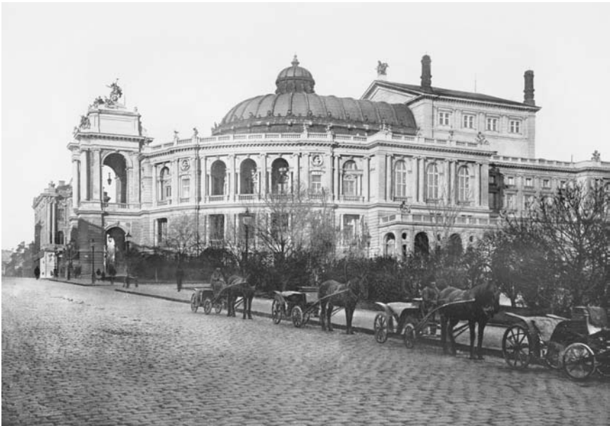
Odesa is filled with historic 19th-century Russian-style architecture, such as this ornate building. (Courtesy Library of Congress)
